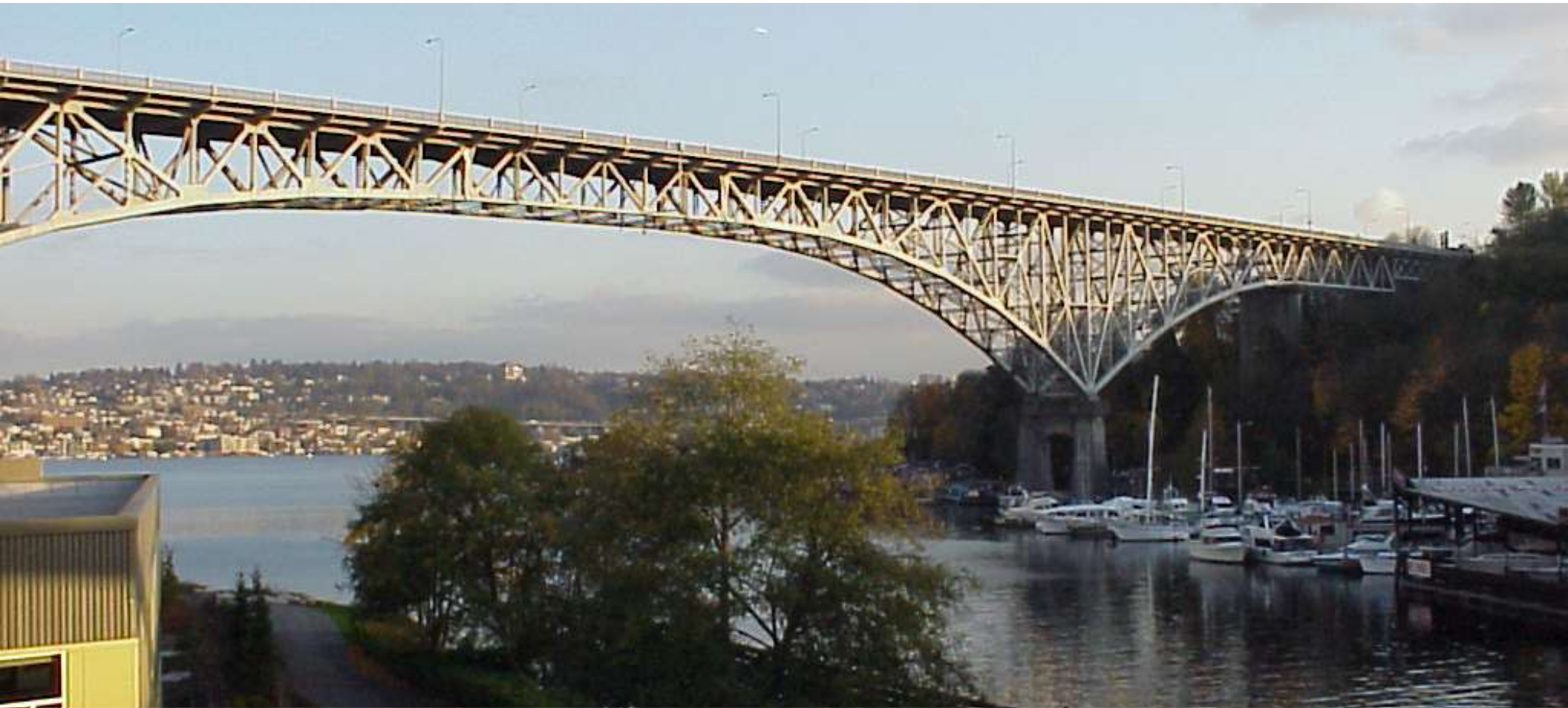
Aurora Avenue Bridge
