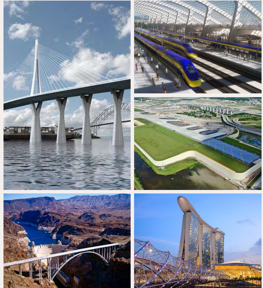
Top Left: New Champlain Bridge (Montreal, Quebec Canada). Top Right: California High Speed Rail (California, USA) Middle Right: New Runway Fort Lauderdale/Hollywood International Airport (Florida, USA). Bottom Left: Hoover Dam Bypass (Clark County, NV & Mohave County AZ). Bottom Right: Marina Bay Sands Integrated Resort (Singapore).
