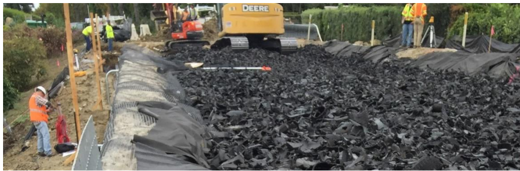
MSTDA Wall Constructed near Montecito, CA in 2019
