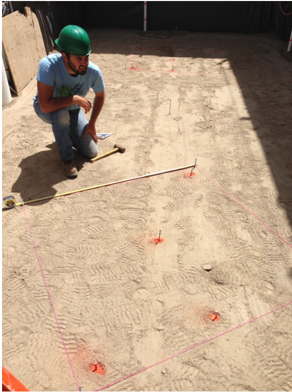
Marking of locations before placement
