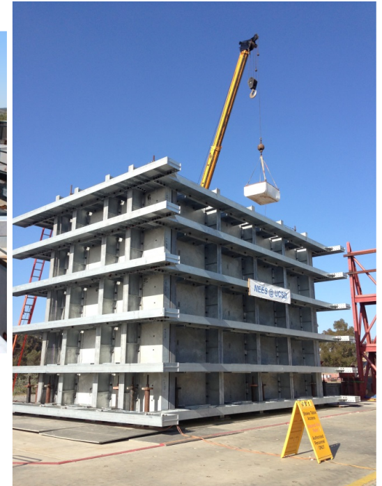
Hopper and crane method (fast and expensive)
