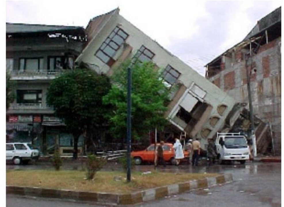
Overturning of building B1 as seen from the North-West after the Kocaeli event. (Photo by Jonathan D. Bray)
