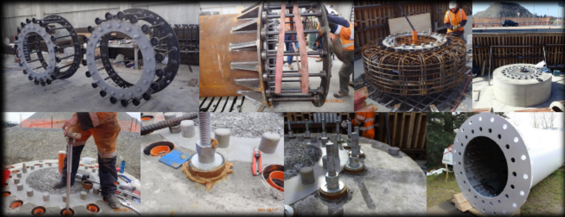
Design detail of bridge piers: steel armoring and dissipators
