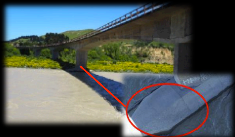
Shear cracking in the piled footing
