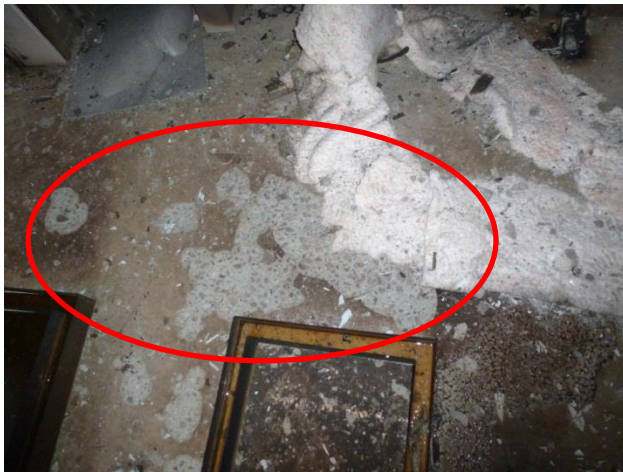
Spalling of concrete slab
