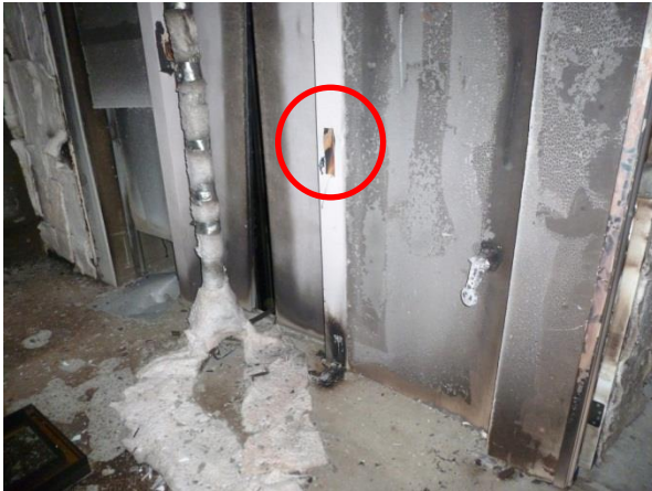
Elevator controls melted
