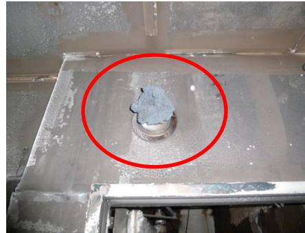
Intumescing of fire stop
