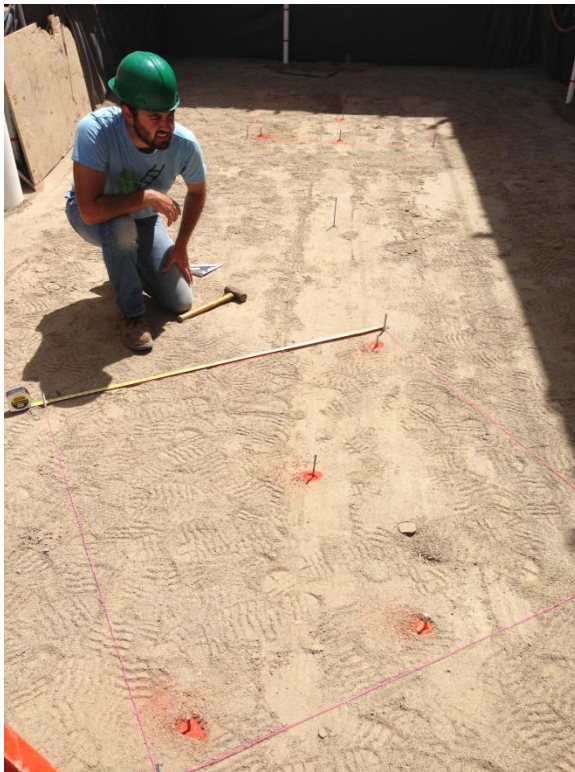
Marking of locations before placement
