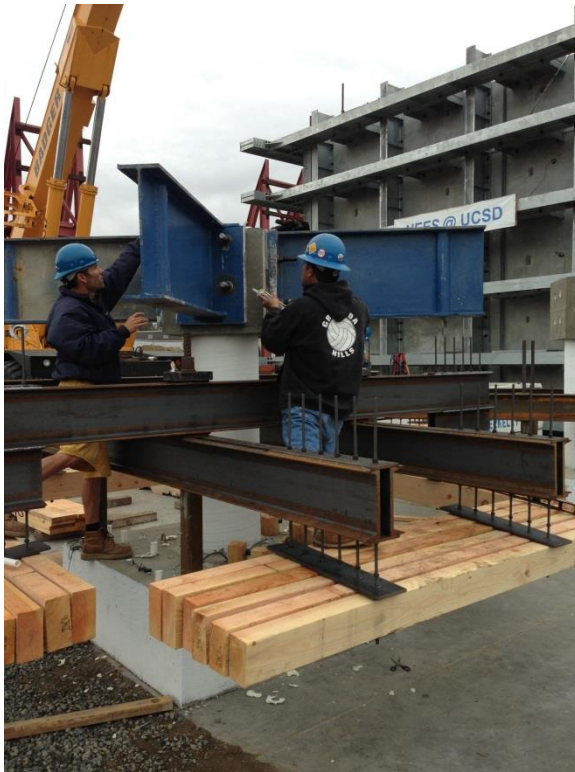
Placement of mass support steel beams
