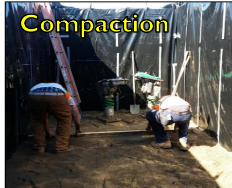
Backfill / Compaction
