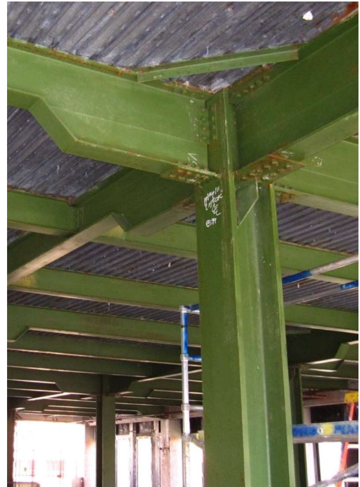
soft-story frame retrofit with a mode-shaping spine
